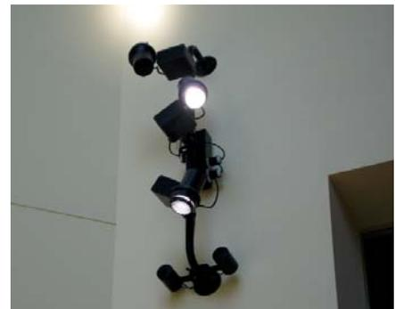
*Standard Oasis Qt™ Emitters painted black and installed in special housing to existing structure*
